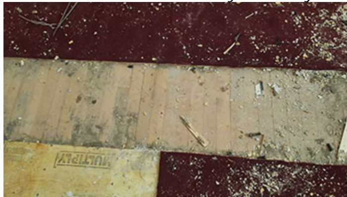
View of the library revealed wood floor
