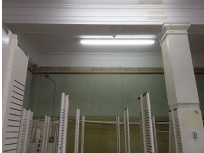
Artwork as shown after the second floor removal
