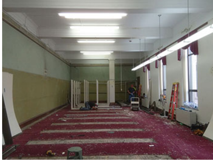
Entire view of the library currently
